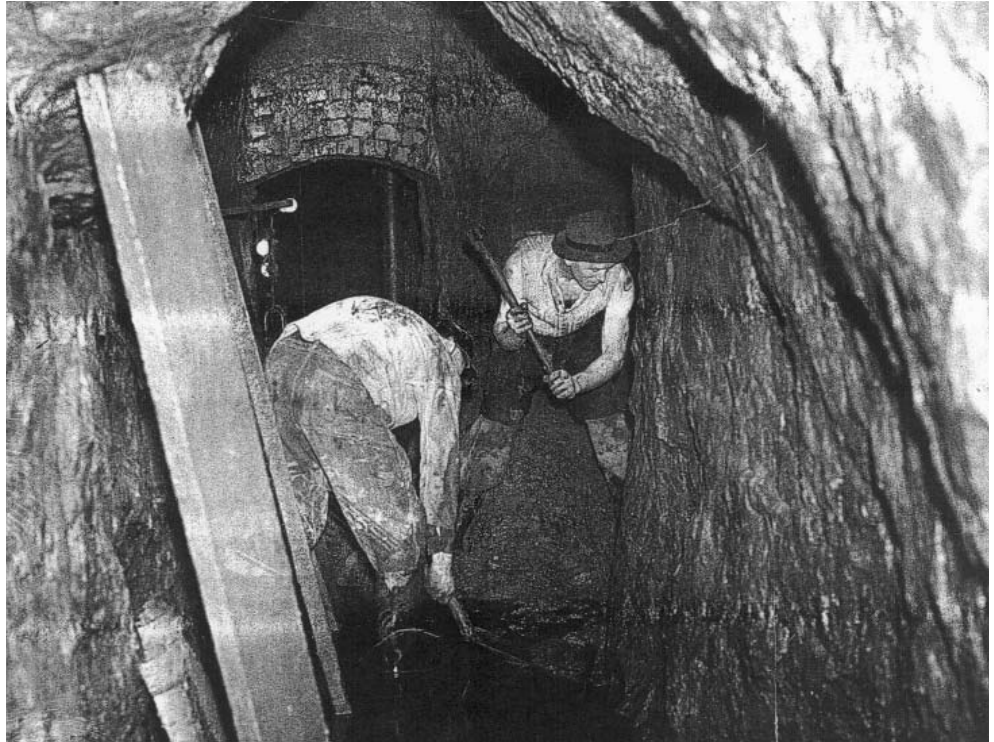
Figure 2. Clearing out the Spa Bath Shaft adits in the winter of 1952-3. (Woodhall Spa Cottage Museum)
